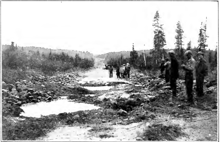
Trans-Canada Highway — Mattawa-North Bay Section — Third Sink Hole After 9 Box Charge.
